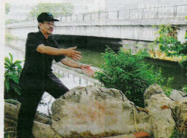
Tunku Ismail Jewfa points to what is believed to be remnants of the concrete structure of the Wan Mohammad Saman Bridge, which was blown up by retreating British troops. In the background is the present bridge.
